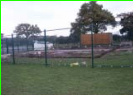
The foundations of our new clubhouse
